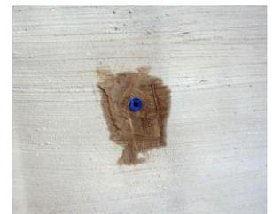
Where fixings have to be made, provisions should be made in advance by drilling oversized holes and plugging with CONSTRUCTION CHEMICALS WATERSEAL, then insert a fixing plug whilst the water seal is still soft, alternatively wait till the waterseal has cured then drill the correct size hole.
