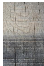
The top half of this old oak beam was cleaned with oxalic acid, the cleaning took less than 3 mins.
