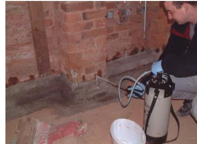
3 Fill boreholes with **ONE SHOT** Injection Cream using a low pressure sprayer, injection cream gun or injection cream cartridge.
