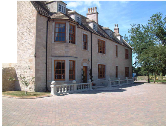
Stretton Hall on the border of Lincolnshire and Leicestershire, refurbished to a high standard using many of Construction Chemicals products. The cellars have been waterproofed using tanking slurry and have been converted into a gym, sauna and plunge pool.
