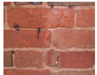
This picture clearly shows areas treated with Façade water repellent.
